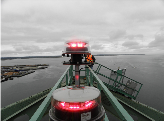
Solar Navigation Lighting System, Astoria-Megler Bridge -Photo courtesy of Oregon Department of Transportation
